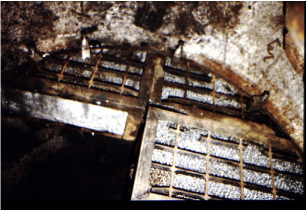
FIGURE 3-20 Installation of replacement mist extractor.
